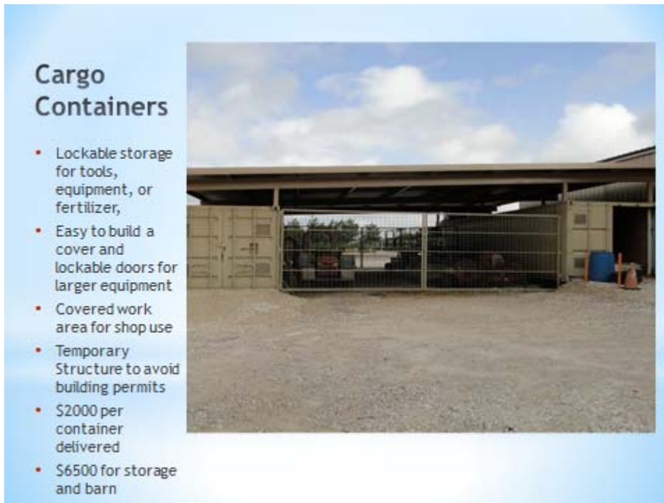
Figure 12. Cargo containers can be utilized as inexpensive building options for shop use, storage and secure office space.
